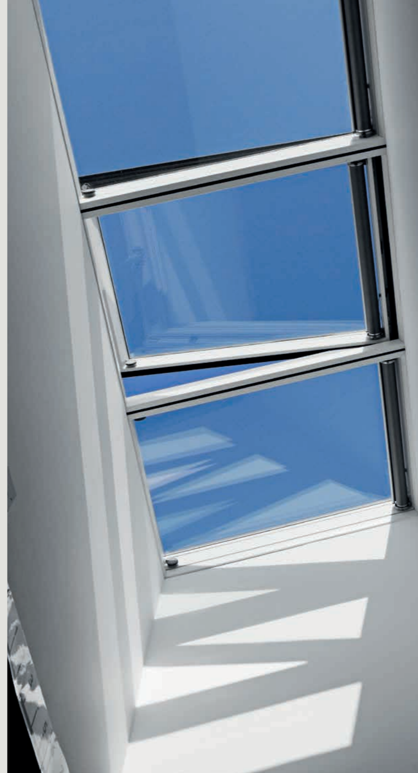
Venting modules provide fresh air and cooling to classrooms and common areas.
